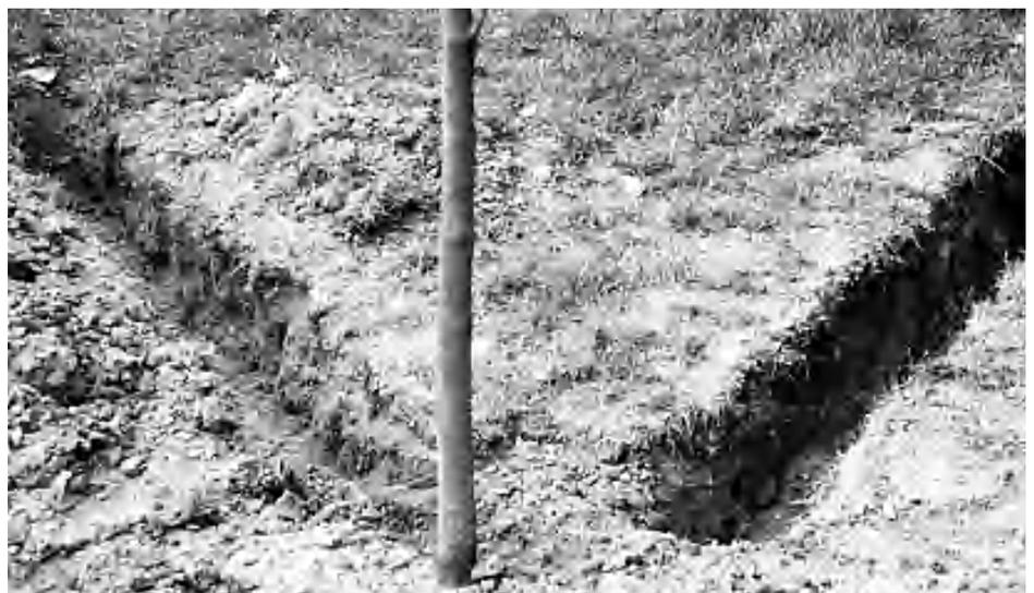
**Fig. 32.** Placing a thin amount of soil over compacted gravel or clay does not allow for good plant growth. The parking lot planter should be well drained and filled with a minimum of 4 feet of fertile topsoil.
