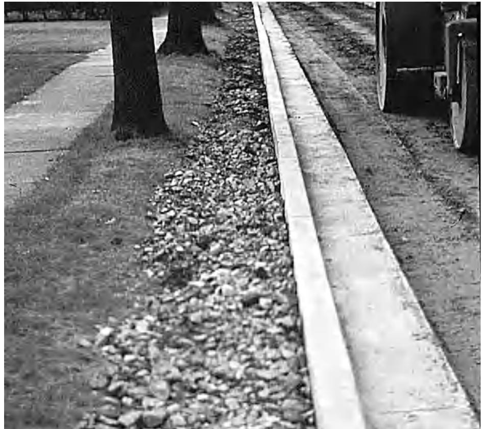
Fig. 20A. Example of an aeration system that can be constructed from PVC piping for use in sidewalks and other plantings. The system can also be used to promote deep watering.
